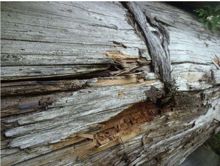
Photo 39: Typical Sap Rot in Cedar Crib Logs
