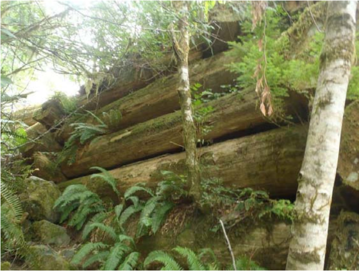
Photo 31: Left Abutment Upstream Wingwall
