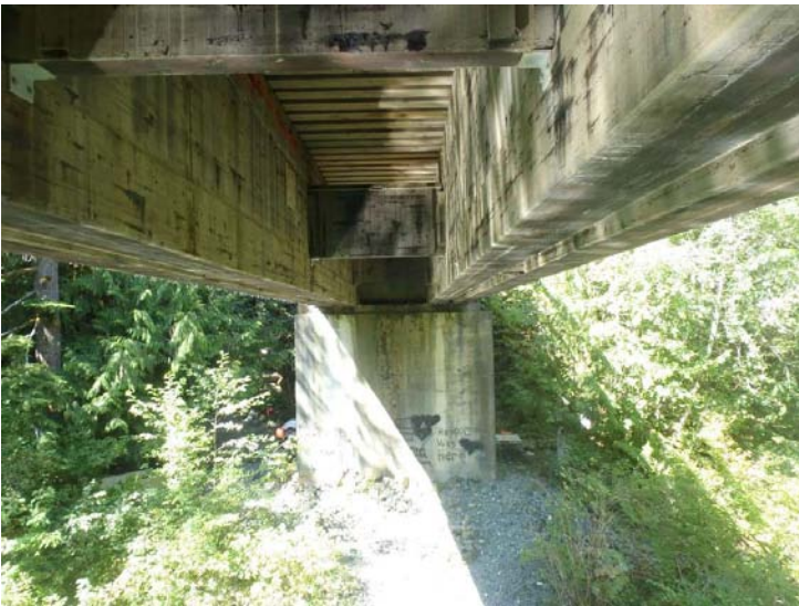
Photo 45: Pier 2 Left Face
