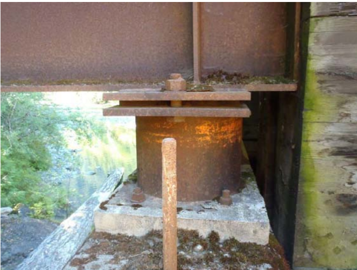
Photo 17: Typical Steel Post Arrangement at Piers
