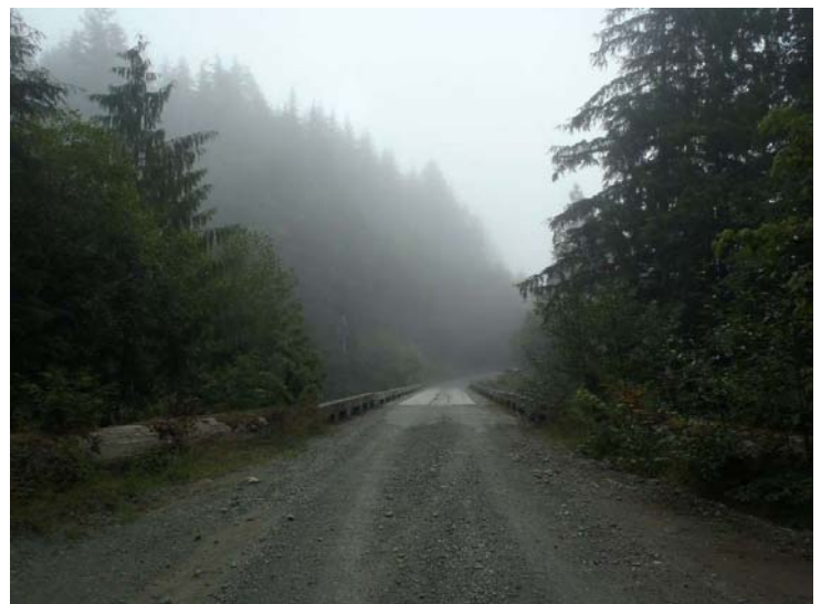
Photo 06: Right Approach Facing Bridge
