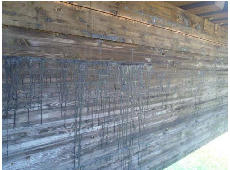
Photo 20: Span 2 Girder 1 Upstream Face
