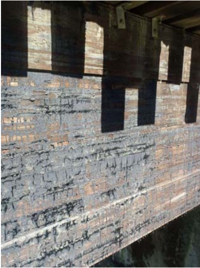
Photo 25: Span 2 Girder 4 Downstream Face
