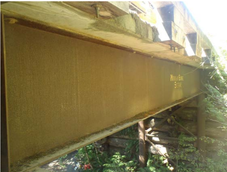
Photo 15: Typical Span 1 & 3 Girder Condition
