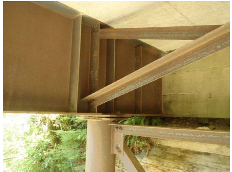
Photo 16: Steel Girders Cantilever Over Steel Columns at Abutments
