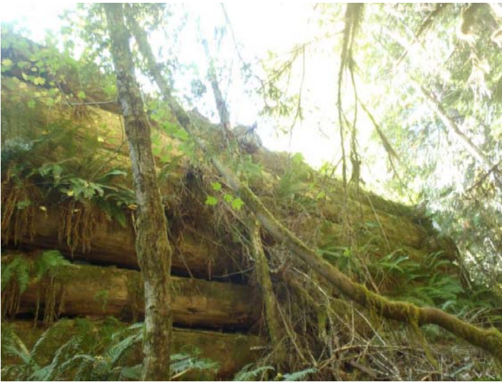
Photo 37: Right Abutment Upstream Wingwall
