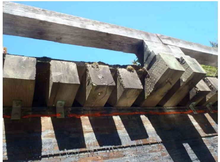
Photo 28: Span 2 Girder 4 Typical Checking in Line with Tie Clips
