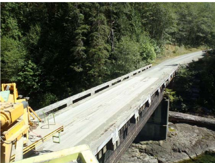
Photo 05: Looking Right Across Bridge
