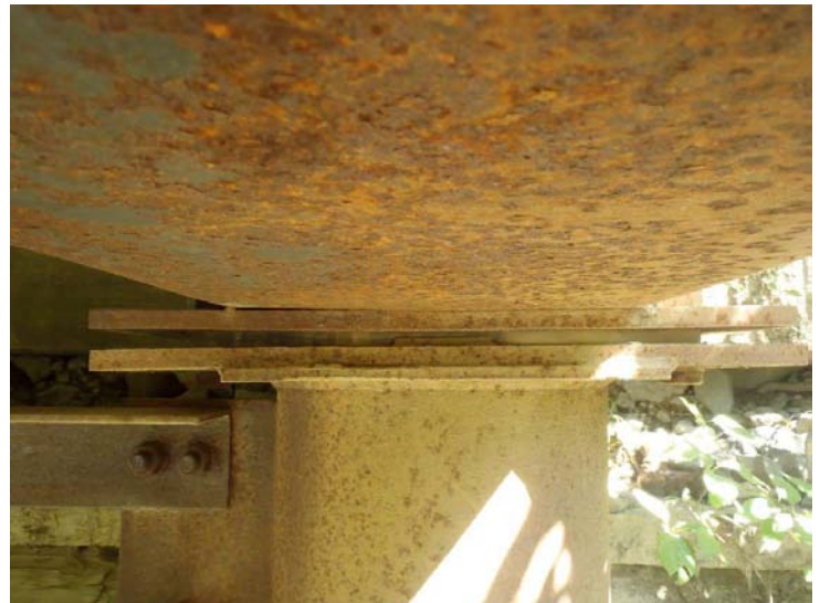
Photo 18: Typical Steel Span Bearing Condition
