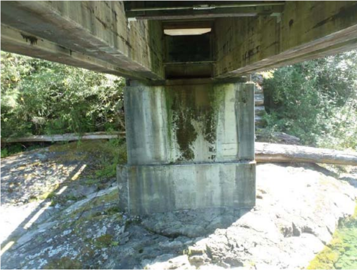
Photo 43: Pier 1 Right Face
