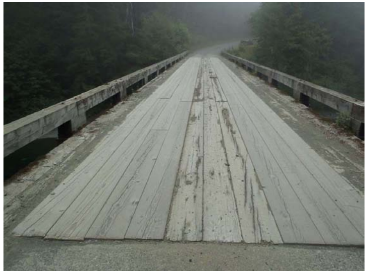
Photo 10: Span 2 Timber Deck Condition
