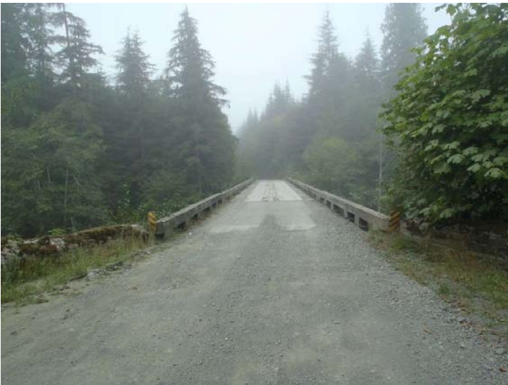
Photo 07: Left Approach Facing Bridge
