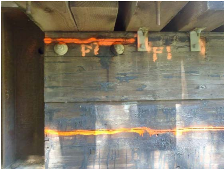
Photo 27: Girder 4 at Pier 2
