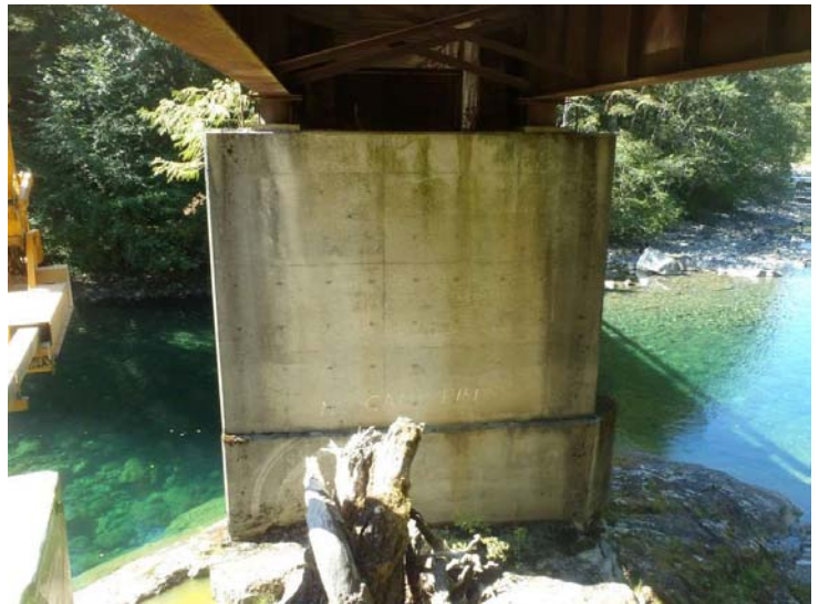
Photo 42: Pier 1 Left Face
