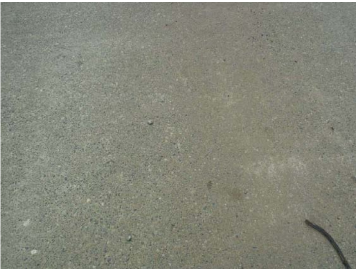
Photo 09: Typical Deck Panel Condition
