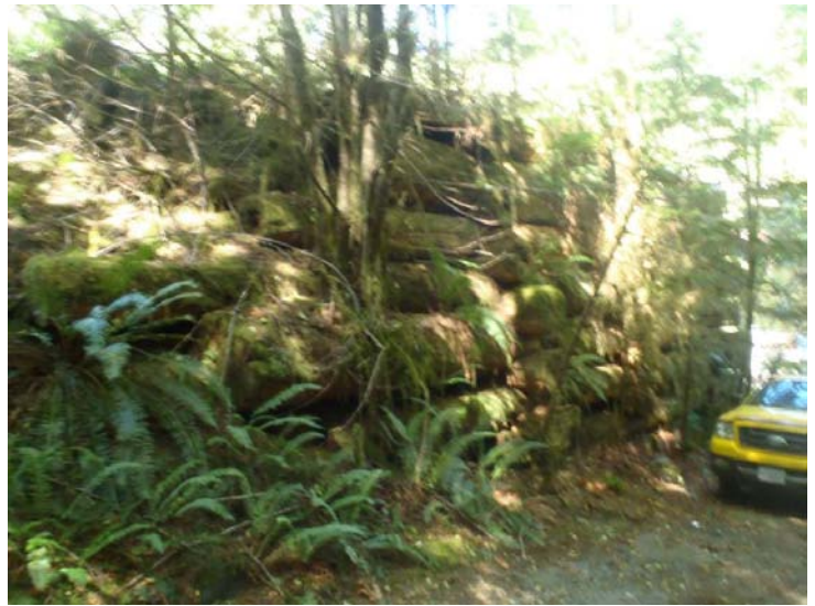
Photo 38: Right Abutment Downstream Wingwall
