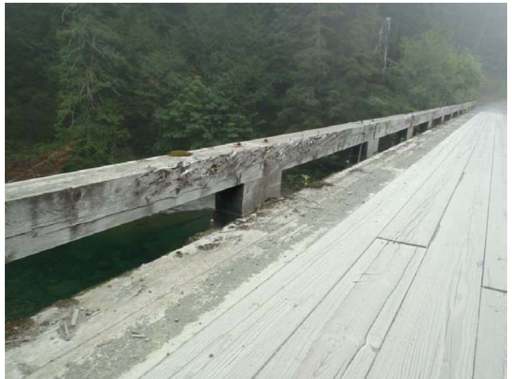
Photo 08: Typical Curb Rail Condition
