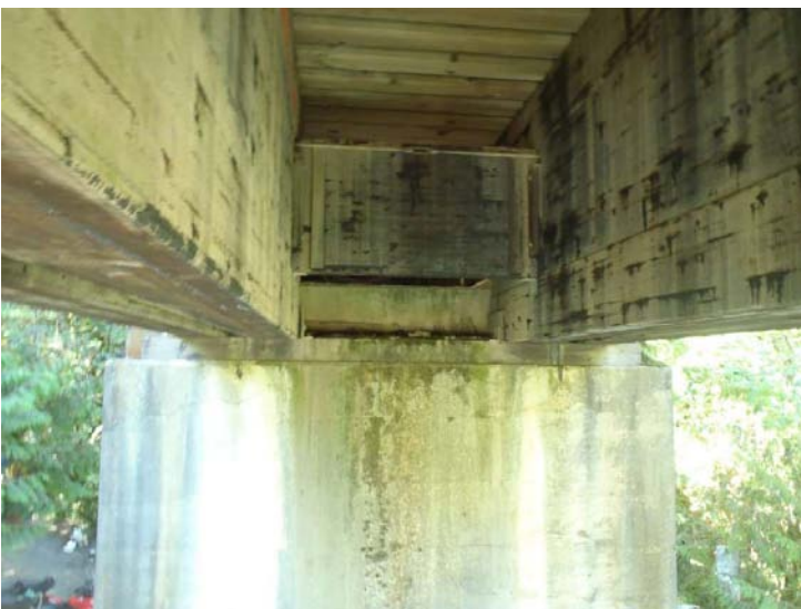
Photo 47: Typical Pier Condition
