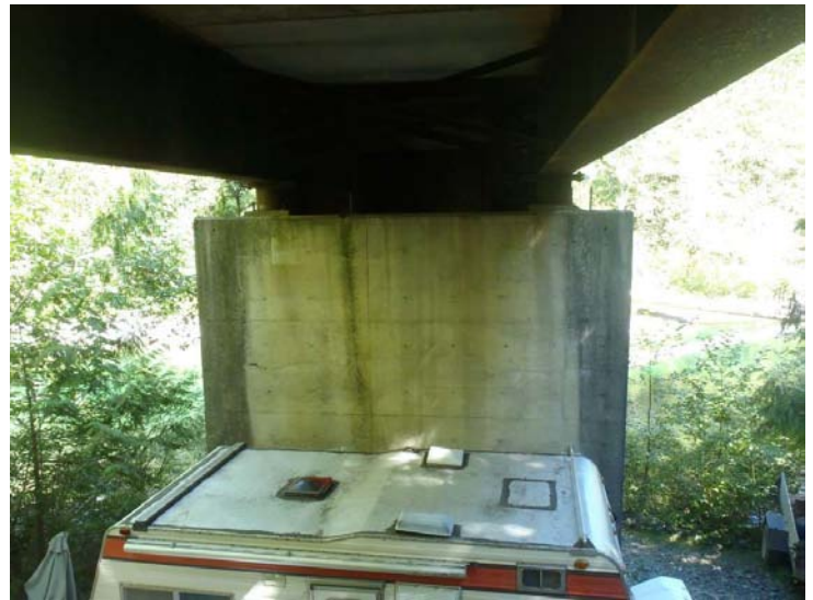
Photo 46: Pier 2 Right Face
