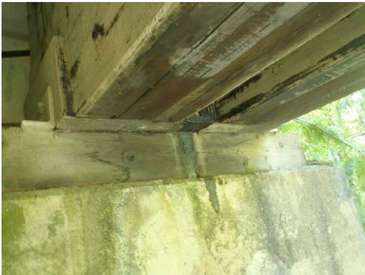
Photo 29: Span 2 Typical Timber Sill and Anchor Detail
